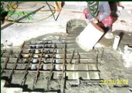
Grouting Beton
