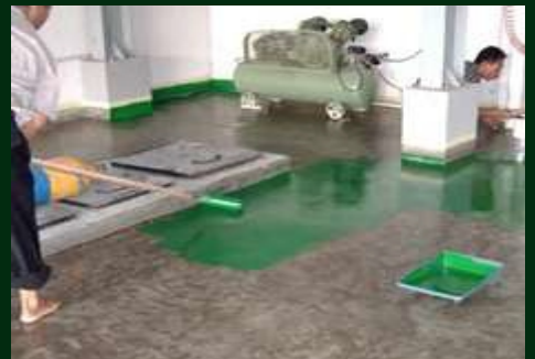
Epoxy Coating Flooring
