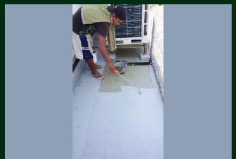
Waterproofing Polyurethane
