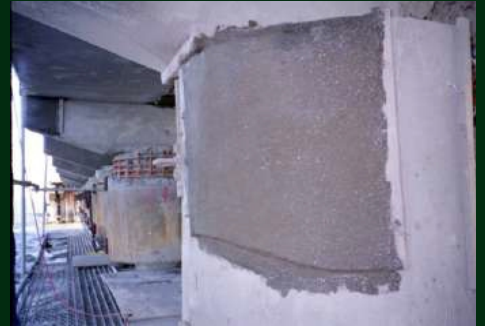
Patching Concrete
